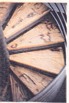
The treads on the spiral staircase in the addition are engineered lumber made of discarded wood scraps left unpainted and unfinished, above. Hand-blown glass pendant lights by Jason Wein, of Cleveland, right, hang on Romex cable.
